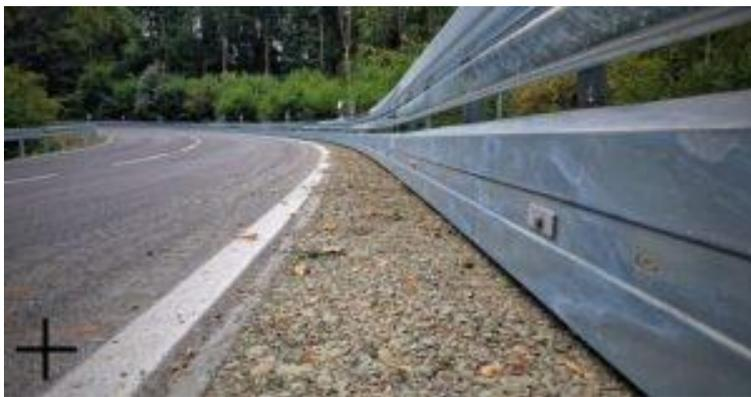
Motorcycle protection on guard rails can be a real life saver (photograph courtesy of PASS+CO).
